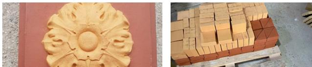
During the cleaning process, yellow stones emerged that had been hidden under layers of dirt over time, revealing beautiful details and floral carvings that served as the basis for producing new stones used to repair the rest of the facade.
